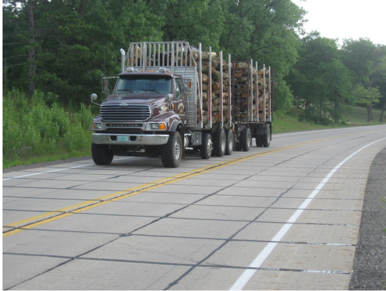
Figure 6a. Wisconsin SJPCP with 4x4 joint spacing. Note the closeness of the wheel loads to the longitudinal joints and corners.
