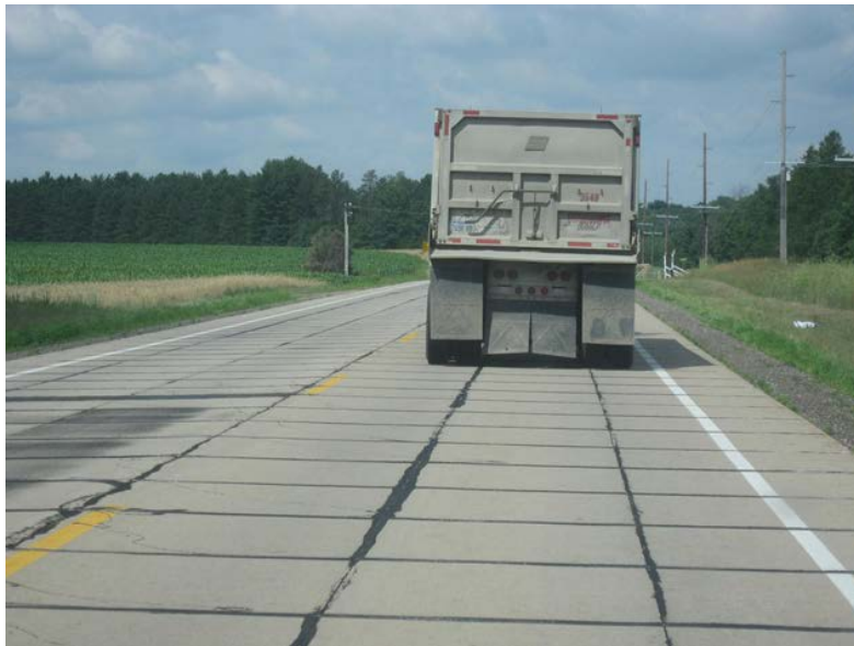
Figure 6b. Wisconsin SJPCP with 4x4 joint spacing. Note that with any lateral wander, the wheel loads will load the slab corners more frequently.
