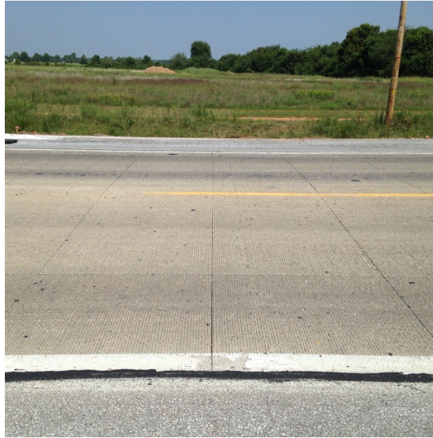
Figure 14. Recent photo of Missouri US 60 after 16 years in service, 4x4 ft joint spacing. (Photo courtesy of John Donahue, MoDOT)
